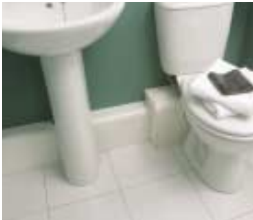
Covering waste pipes.
