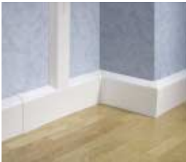
Covering heating pipework.
